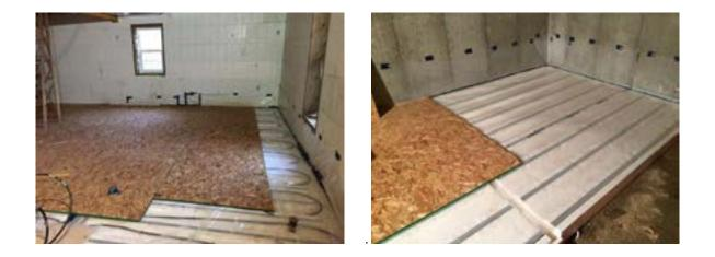
Sheeting of the floor runs perpendicular to the stud lines of the sections, and is attached using approved supplied screws on 12 inch centers through the deck into the section steel studs. Sheets are butt jointed on studs at the short ends and tongue and groove connected don the long edges, the identical process of installing sheeting on any floor joist system used in residential construction.
