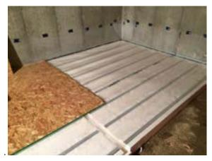
Sheeting of the floor runs perpendicular to the stud lines of the sections, and is attached using approved supplied screws on 12 inch centers through the deck into the section steel studs. Sheets are butt jointed on studs at the short ends and tongue and groove connected don the long edges, the identical process of installing sheeting on any floor joist system used in residential construction.
