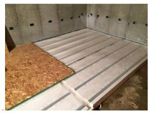
Sheeting of the floor runs perpendicular to the stud lines of the sections, and is attached using approved supplied screws on 12 inch centers through the deck into the section steel studs. Sheets are butt jointed on studs at the short ends and tongue and groove connected don the long edges, the identical process of installing sheeting on any floor joist system used in residential construction.
